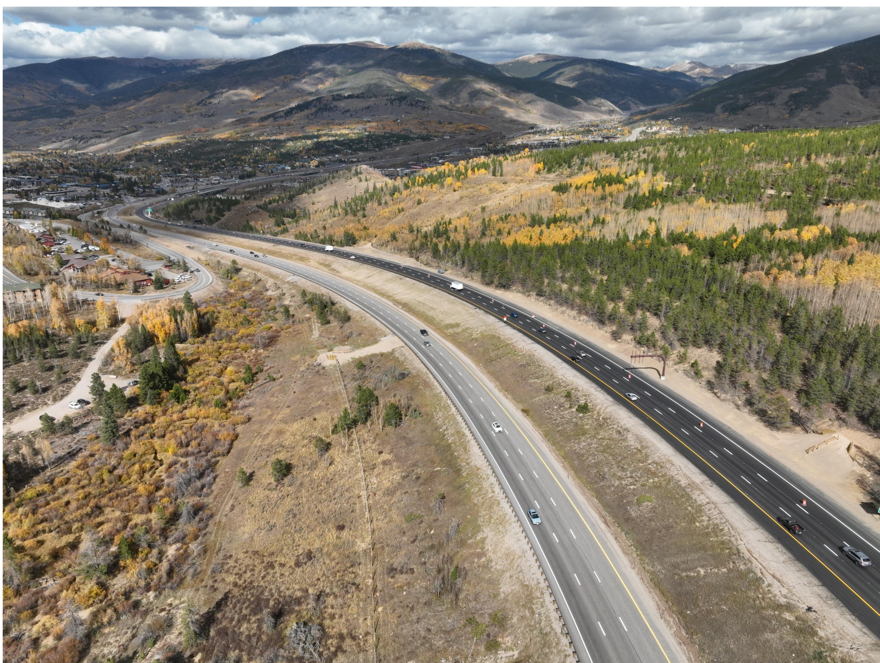
I-70 EASTBOUND AUXILIARY LANE LOOKING TOWARDS SILVERTHORNE/DILLON (SEPT 2023)
